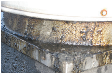
Exhaust systems must be FOG free.
